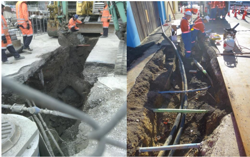
Figure 2: Examples of some “Unexpected” Shallow Ground Services in Section A
