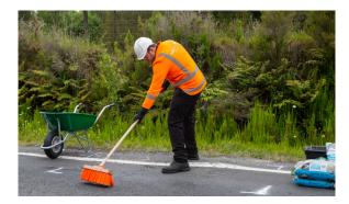
> Remove loose material, sweep the surface, ideally surface should be dry.
