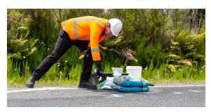
Remove loose material, sweep the surface, and ideally the surface should be dry
